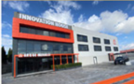
Innovation House R&D Center
